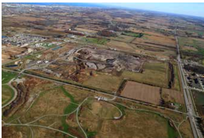
Aerial view of SCRF and surrounding area.
